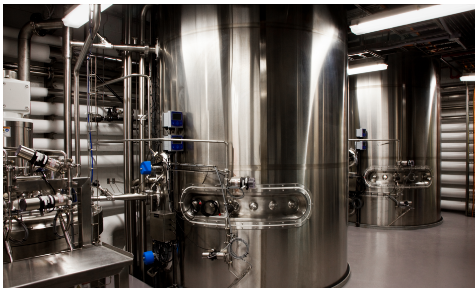
Two 17,000-L fermenters located in the fermentation hall at BioVectra’s Windsor, Nova Scotia, facility
